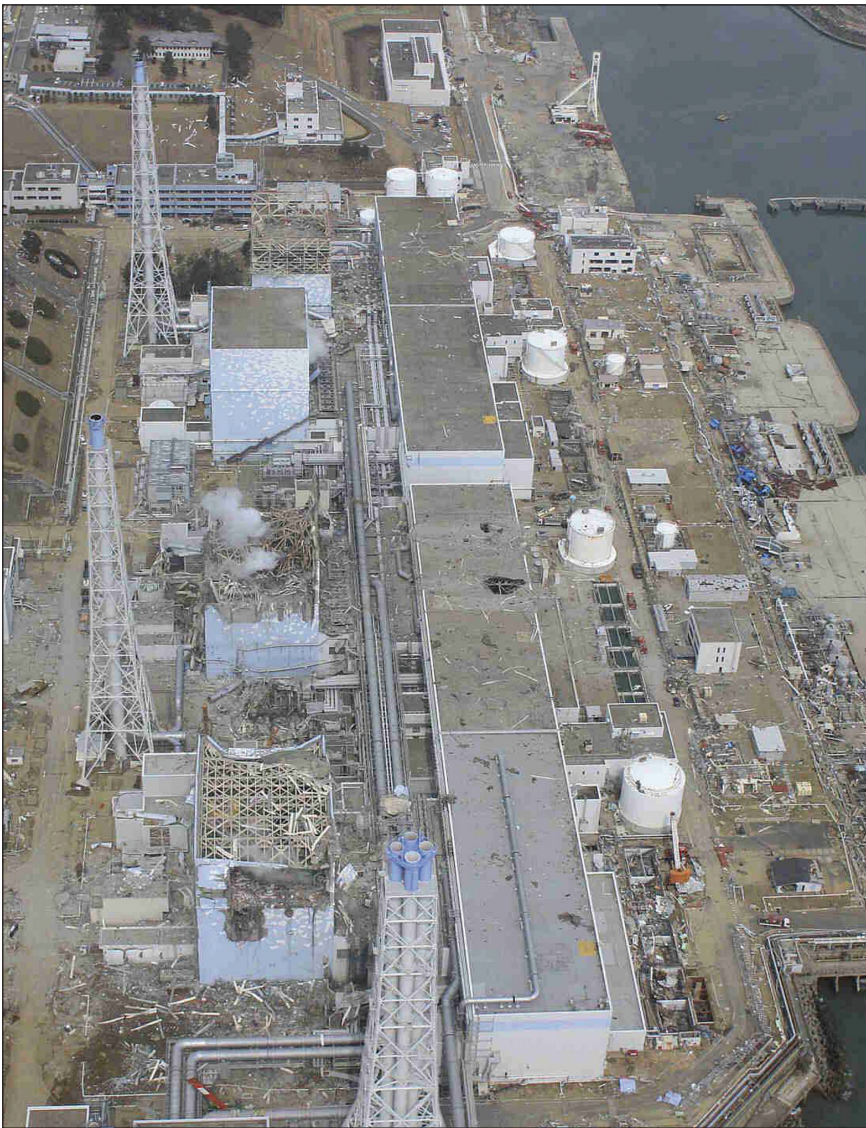
FIGURE FUK 1 Aerial image of the Fukushima nuclear power plant complex after the initial explosions in March 2011. SOURCE: Copyright Air Photo Service Co. Ltd., Japan.
